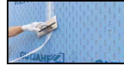
Application Watec ST - bandes de calicot
